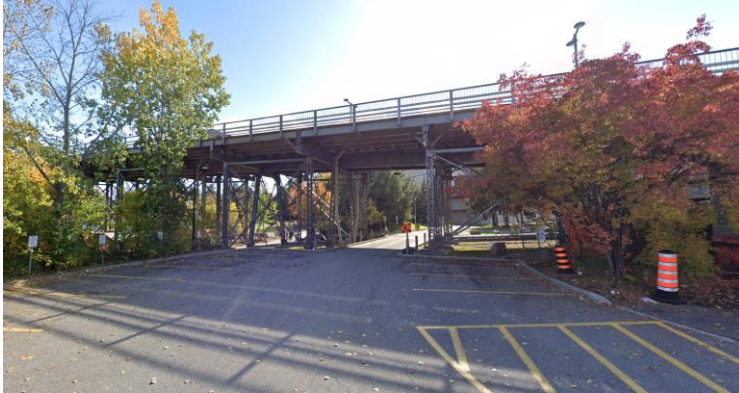
Figure 6 : Existing conditions under the bridge on Gatineau side
