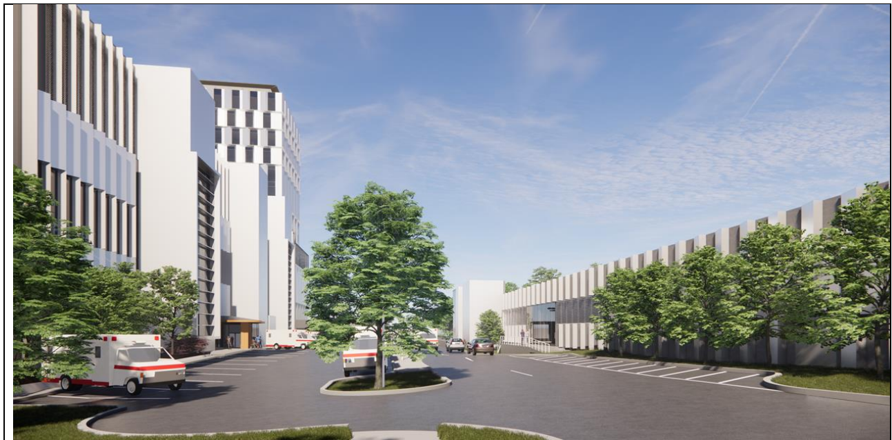
Figure 4: Looking east – Central Utility Plan on the right
