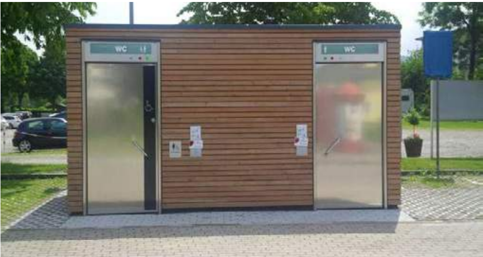
Fig. 119 Toilettes publiques Source: cellcode.us/quotes/ada-design-bathroom-public-compliant.html
