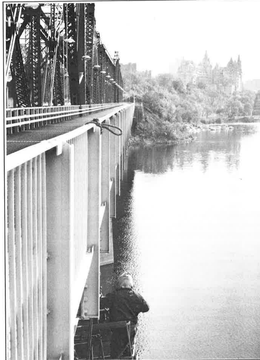
Inspection, Alexandra bridge with Chateau Laurier and Rideau Canal locks in background.
