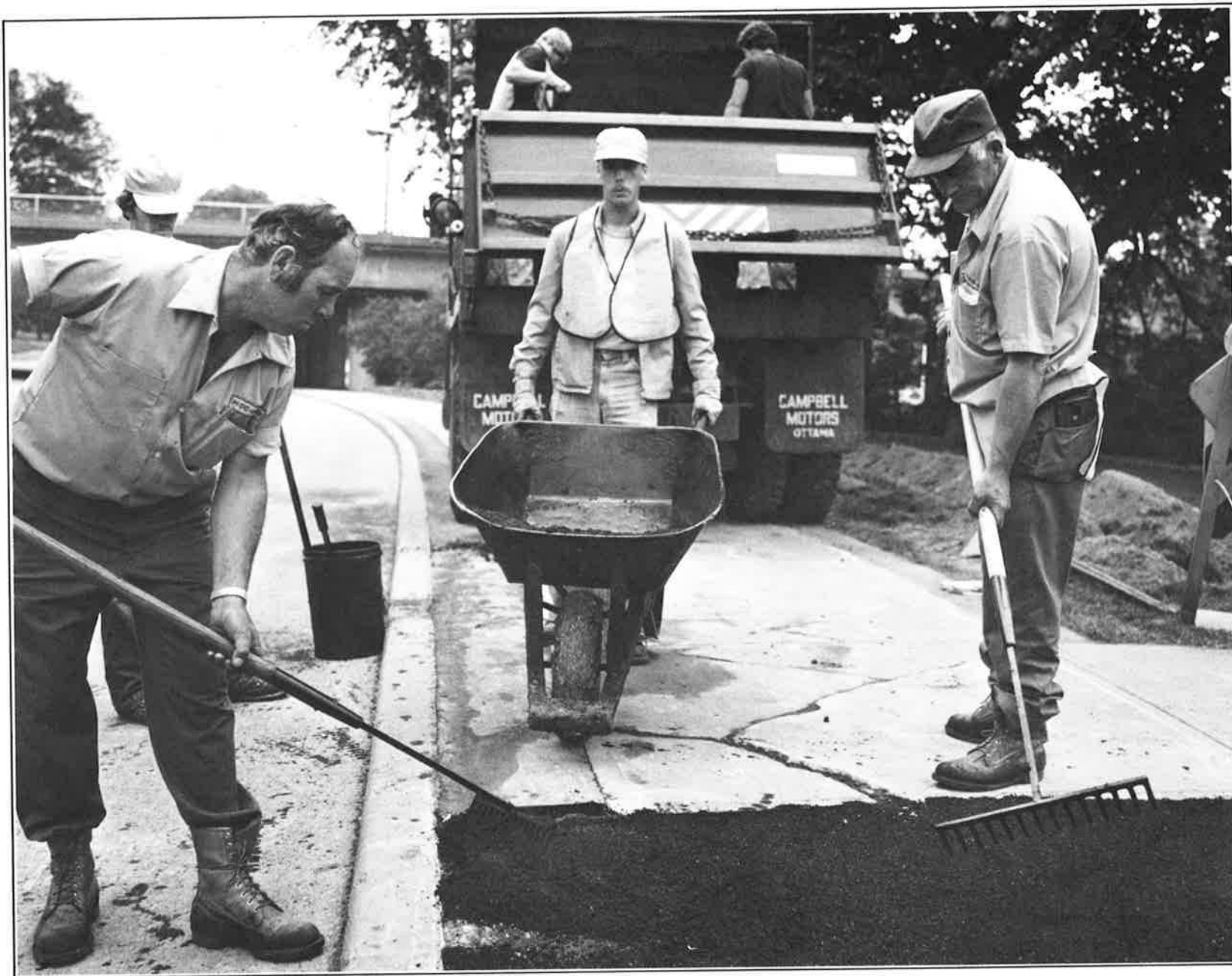
Covering the cracks.
