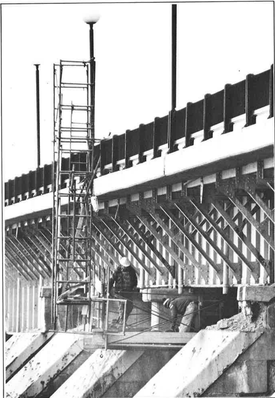
Major repairs begin on 50-year old Champlain Bridge.
