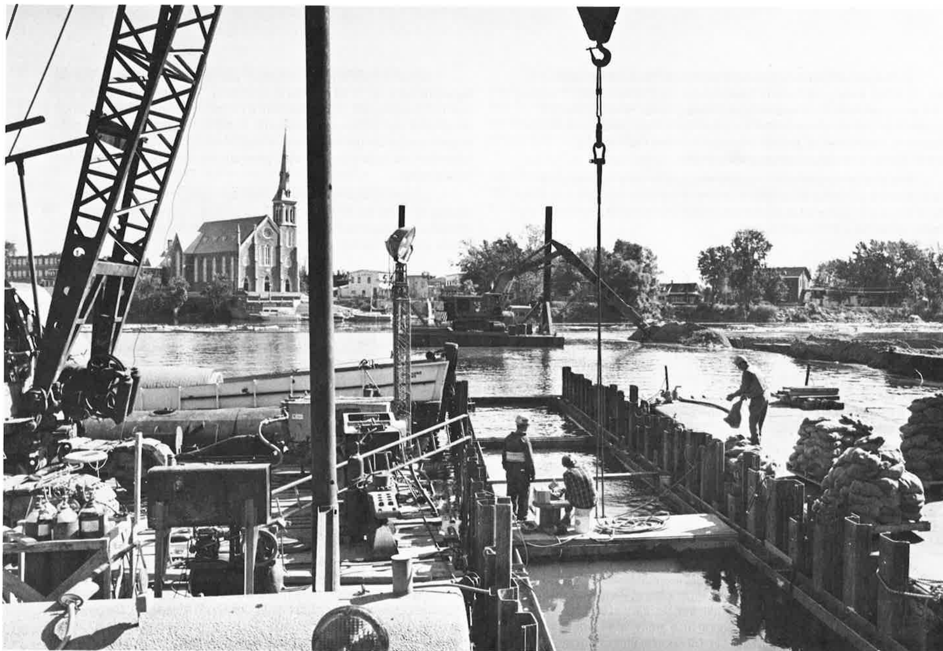
A new trunk sewer system for the Quebec part of the National Capital Region crosses the Gatineau River. The NCC pays one-third of the cost.
