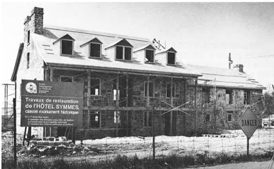
The Symmes Hotel in Aylmer is being restored with the aid of an NCC grant and architectural advice.
