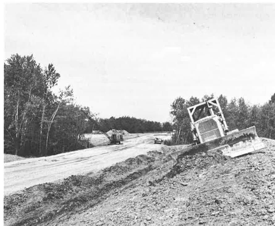
The eight-kilometre Eastern Driveway begins to take shape. It is being built by the NCC on the south bank of the Ottawa River east of Rockcliffe as a scenic entrance into the Capital.
