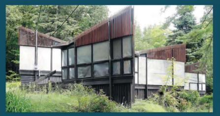
The Strutt House, a recognized federal heritage building, is one of the Capital's most significant homes. The post-war modern residence features the first hyperbolic paraboloid roof in Canada and multi-level wooden facades with pressed concrete. Perched atop a two-level site amongst trees and a rocky ridge, the former home of Canadian architect James Strutt is a private oasis at the edge of the Gatineau Park.
