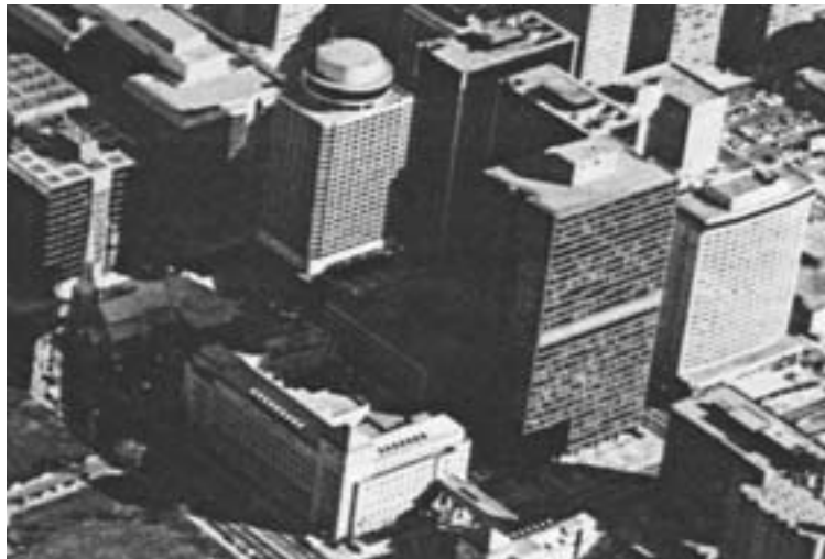
Figure 10: Aerial View of Place de Ville (Ottawa Views, 1993)
