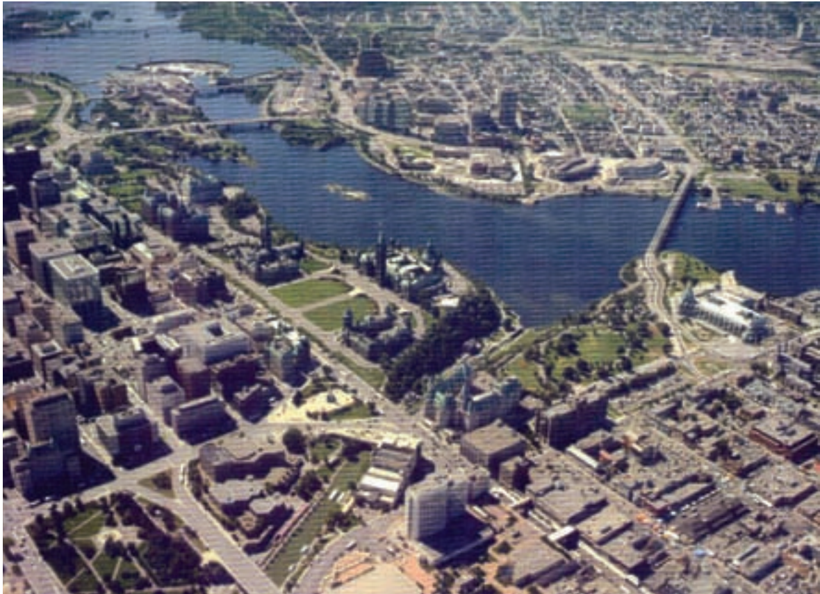
Figure 22: Aerial View of the "Central Capital Landscape"
