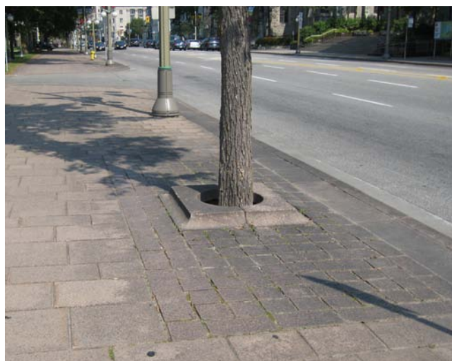
Granite paving and precast concrete collar on Wellington Street
