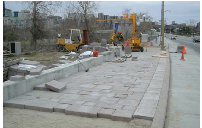
Concrete unit paving during construction
