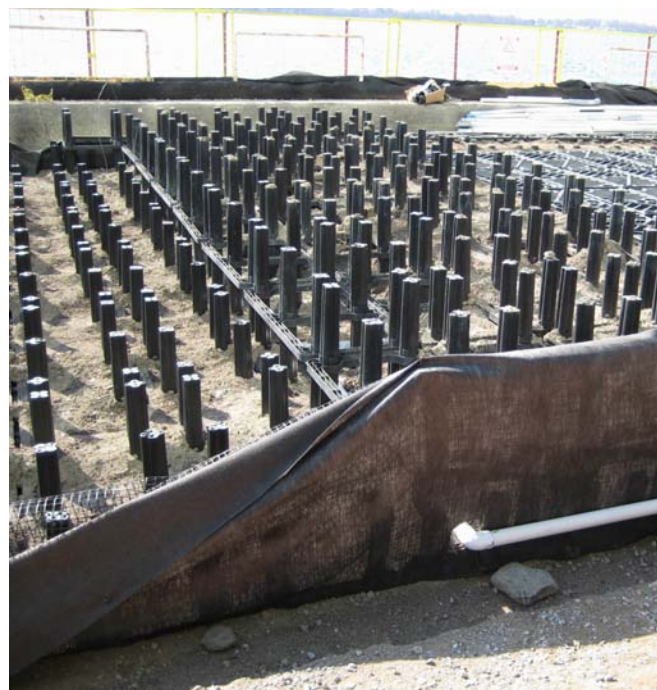
Soil Cells: Improved tree planting technology
