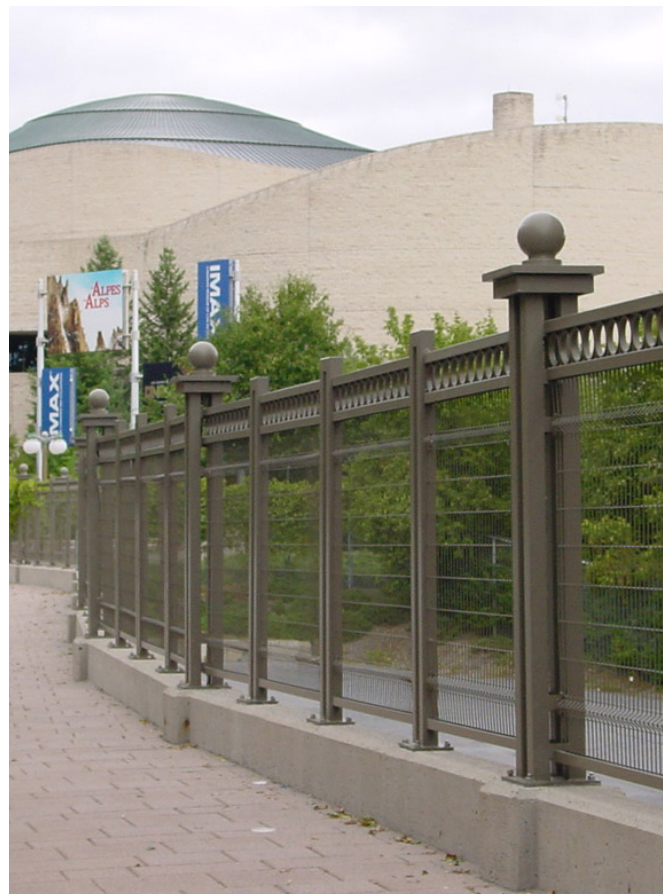
Metal fence: rue Laurier
