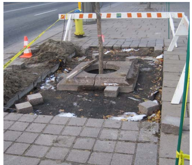
Tree pit repair
