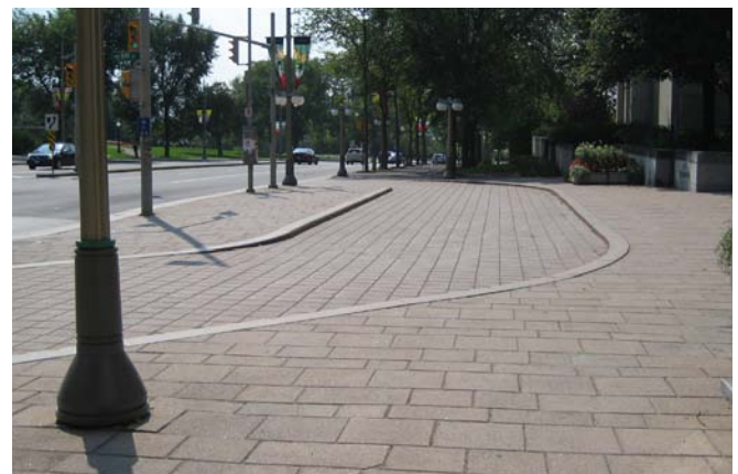
Concrete unit paving on Wellington Street
