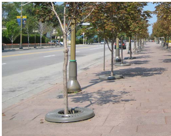
Tree pit paving and metal collar: the first phases of the Boulevard
