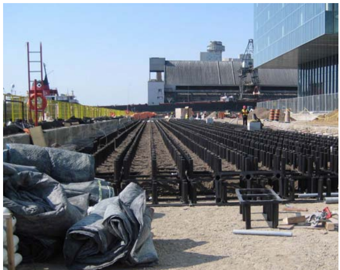
Soil cells being installed on the waterfront in Toronto
