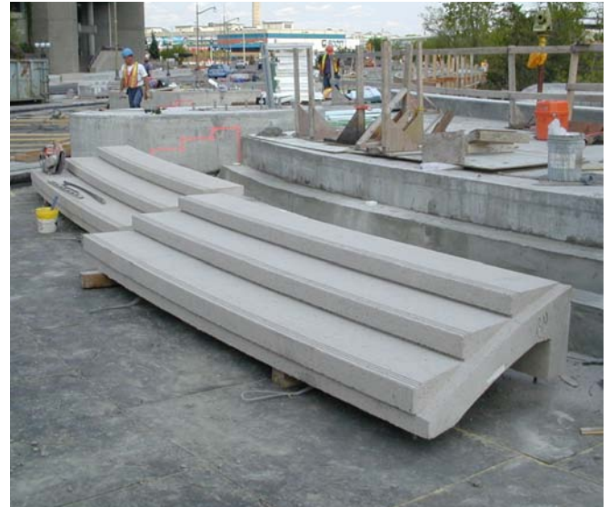
Precast concrete stair during Installation
