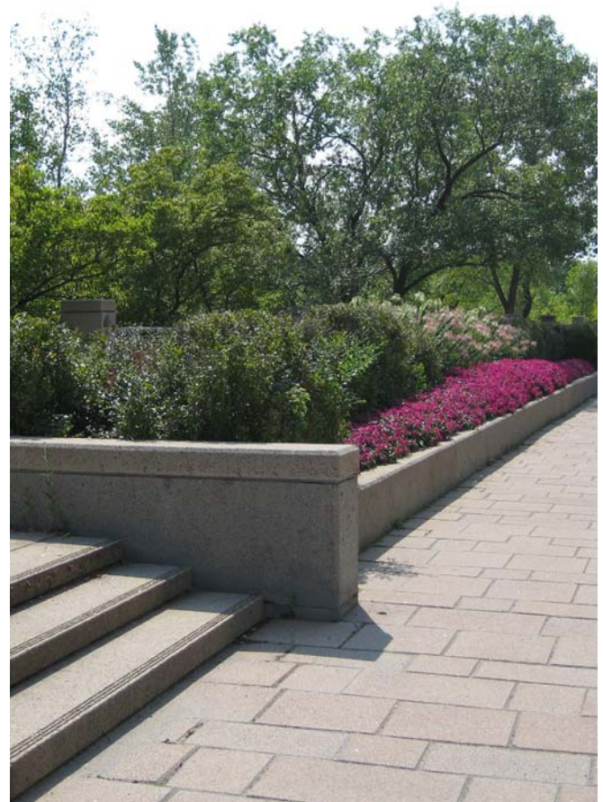
A typical combination of poured-in-place and precast concrete
