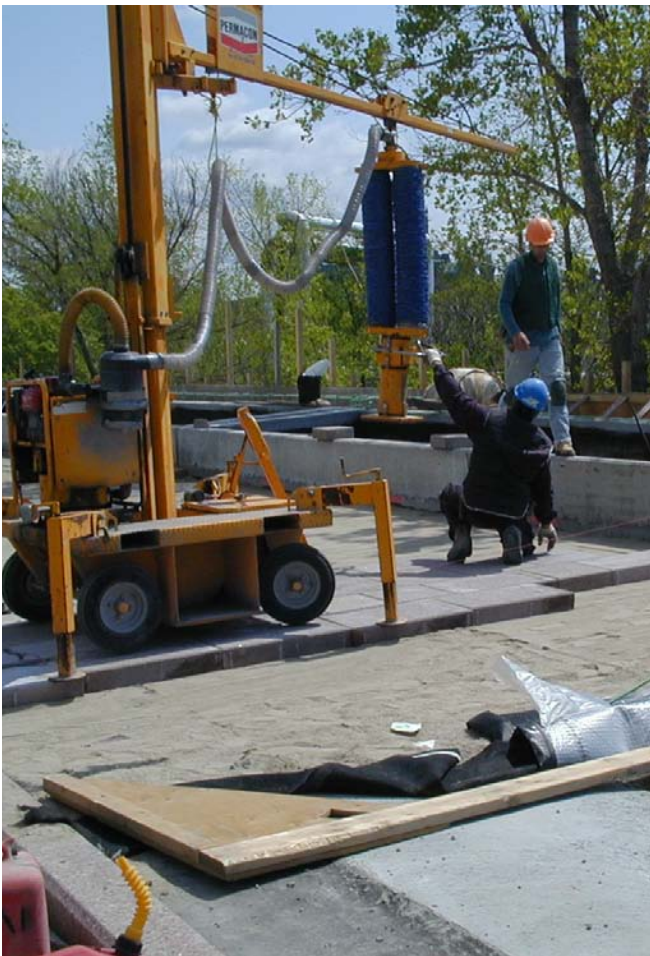
Rue Laurier under construction, 2000
