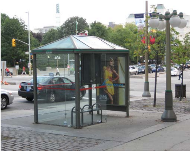
Bus shelter: Elgin Street
