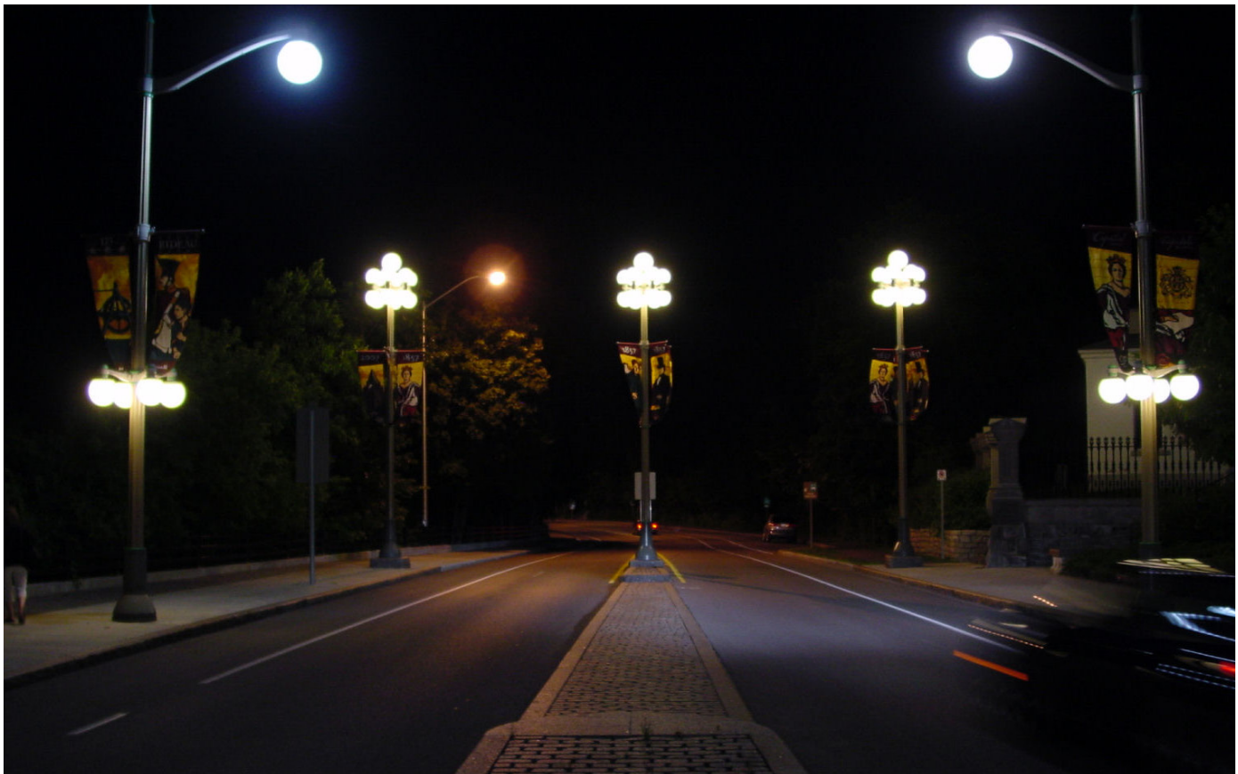
Sussex Drive: Threshold Lights forming the gateway at the northern terminus
