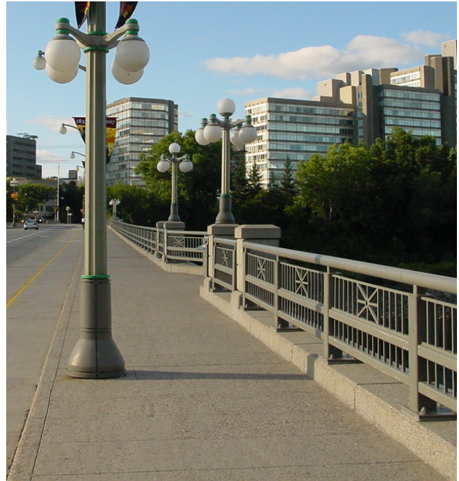
Metal bridge railing: Portage Bridge
