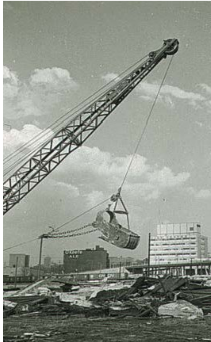
Figure 6 | LeBreton Flats demolition and clearance.
