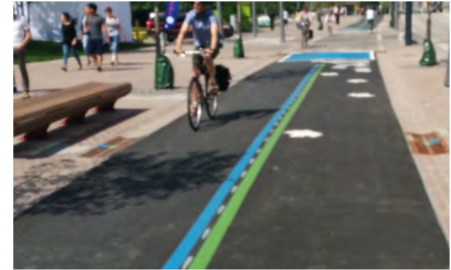
Example of branded pathway centre line along the Great Lakes Waterfront Trail, Toronto, Ontario (see image credits, p.173).
