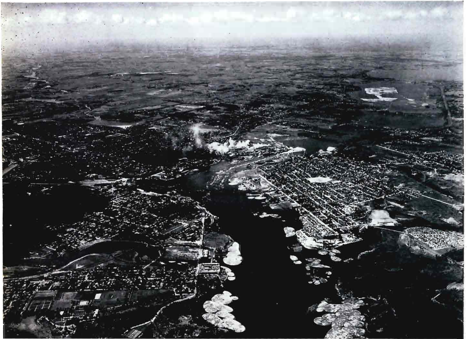
AERIAL VIEW OF THE CITIES OF OTTAWA AND HULL. THE REGION OF THE CAPITAL IS ENHANCED BY THE WIDE SWEEP OF THE OTTAWA RIVER. NOTE, IN THE CENTRE, THE CHAUDIERE FALLS AND PARLIAMENT HILL OVERSHADOWED BY THE SMOKE OF INDUSTRIES
