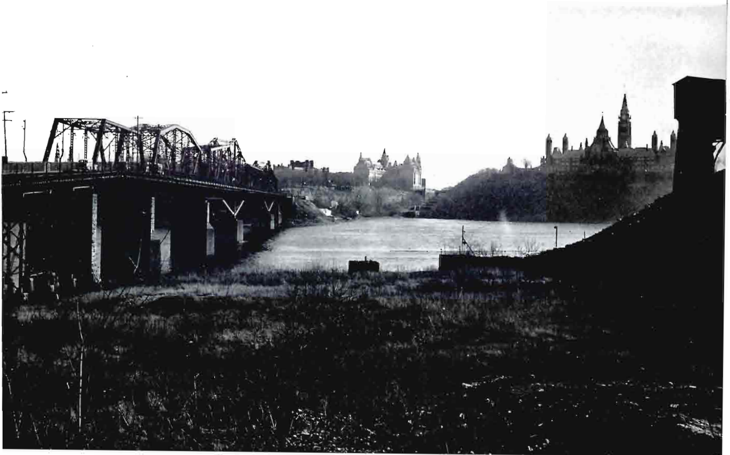
INTERPROVINCIAL BRIDGE VIEWED FROM HULL
