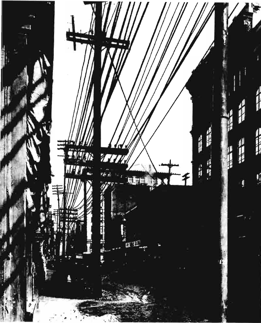
NOTRE DAME STREET, MONTREAL, BEFORE REMOVAL OF PUBLIC UTILITY ELEMENTS
