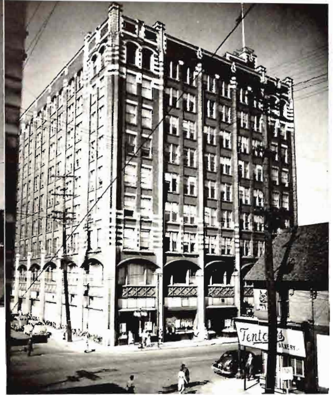
64 THE JACKSON BUILDING IS ONE OF SEVERAL COMMERCIAL STRUCTURES occupied by Government Departments. This building, located on a commercial street, was expropriated in 1940 by the Government to meet wartime needs.
