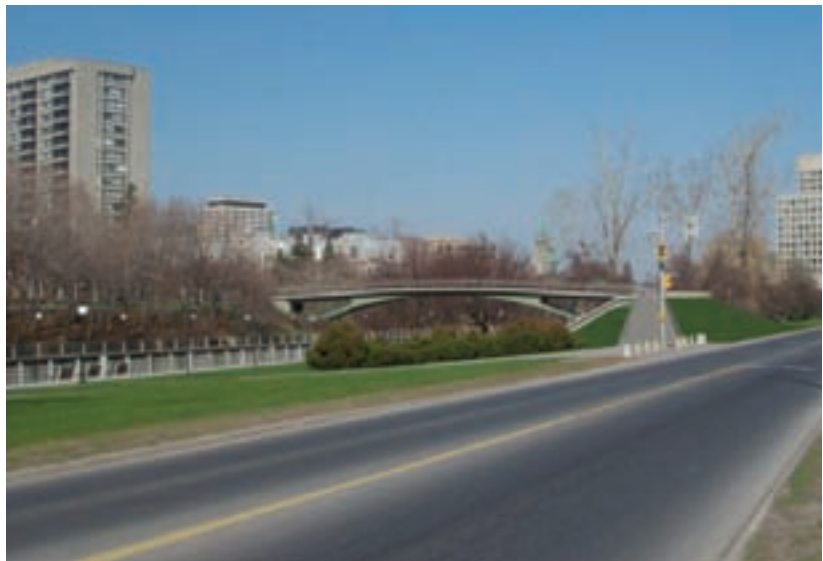
Figure 133: Photo visualization of the Rigid Frame Bridge (Double Leg) from Colonel By Drive
