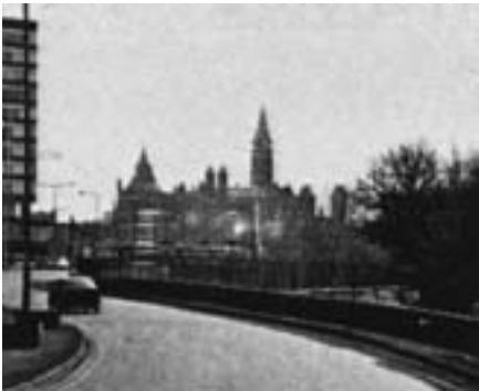
Figure 74: View from Boul. Alexandre-Taché, in Gatinau (formerly Hull)
