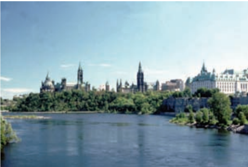
Figure 73: View from the Portage Bridge
