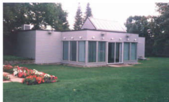
Pool Building (photo NCC 1998)
