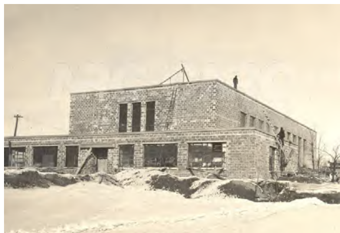
FIGURE 56. CONSTRUCTION DE M-14, 1941 Source : NRC digital depository
