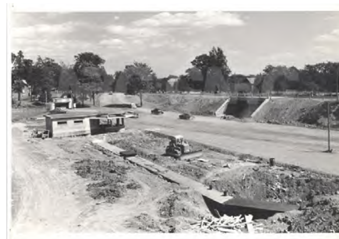
FIGURE 57. VIADUC, 1953 Source : NRC digital depository
