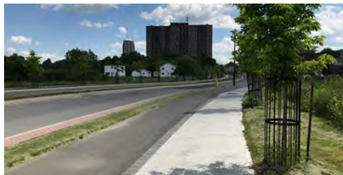
FIGURE 23. WANAKI ROAD SIDEWALK AND BIKE LANE Source: Stantec
