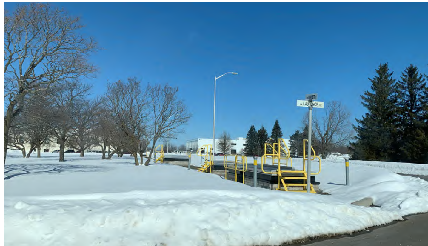
FIGURE 122. PHOTO OF THE HATCH COVERS WITH ACCESS STAIRS AND RAILINGS OF THE ENERGY CORRIDOR Source: Stantec
