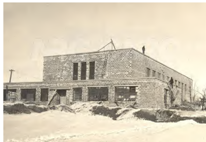
FIGURE 56. M-14 CONSTRUCTION, 1941 Source : NRC digital depository
