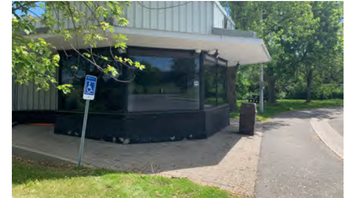
FIGURE 36. LITTER RECEPTACLE AND INTERNATIONAL SYMBOL OF ACCESS NEAR M-1 (GUARD HOUSE) Source : Stantec
