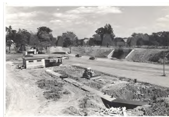
FIGURE 57. OVERPASS, 1953 Source : NRC digital depository
