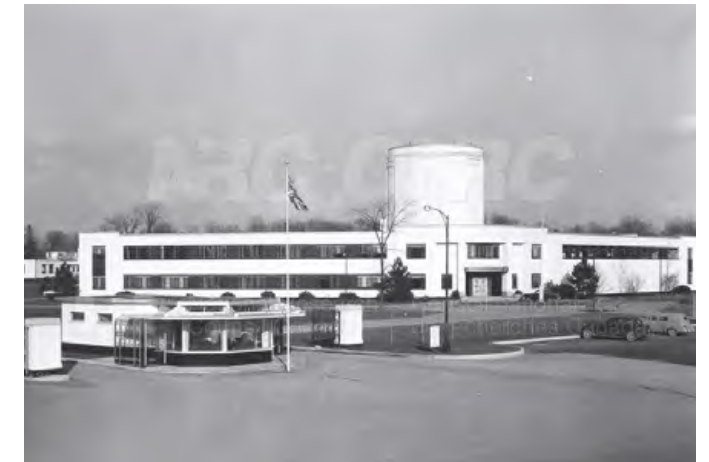
FIGURE 58. NEW GATE, 1955 Source : NRC digital depository
