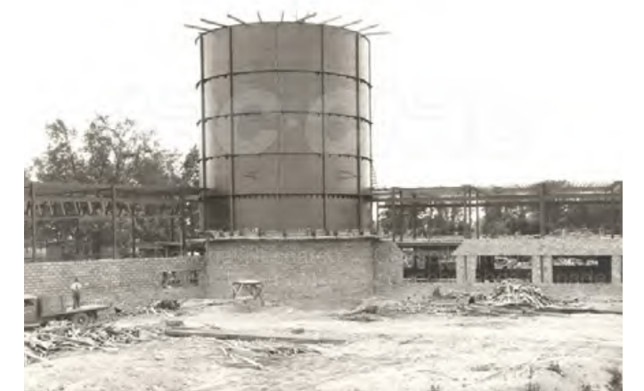
FIGURE 55. M-2 CONSTRUCTION, 1940 Source: NRC digital depository
