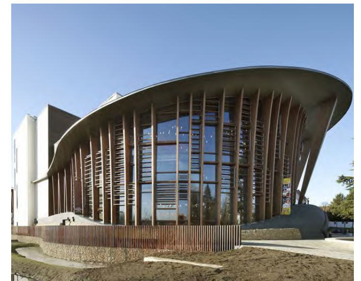
FIGURE 169. PRECEDENT IMAGE FOR THE REAR ADDITION TO M-55, AYLESBURY WATERSIDE THEATRE, LONDON, UK Source: Suzie Bridges Architects
