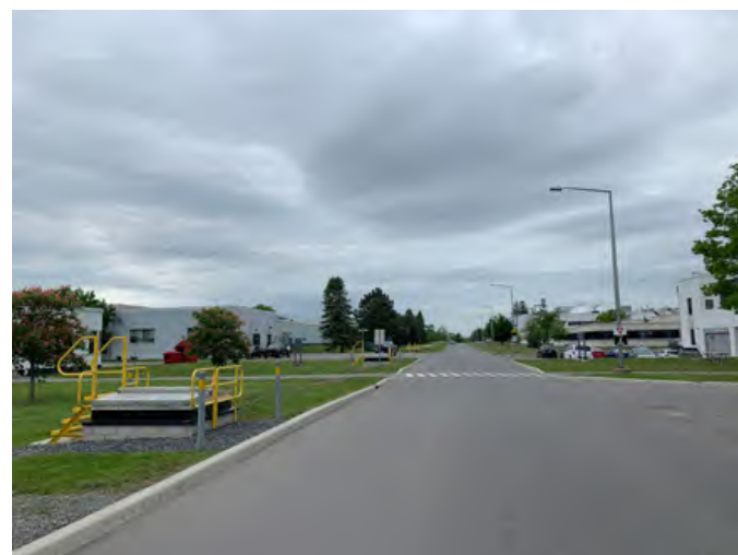
FIGURE 20. MONTREAL ROAD, TOWARDS NORTH, NEAR BUILDING M-7 Source : Stantec
