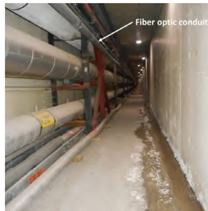
FIGURE 65. TYPICAL TUNNEL SECTION Source : Stantec
