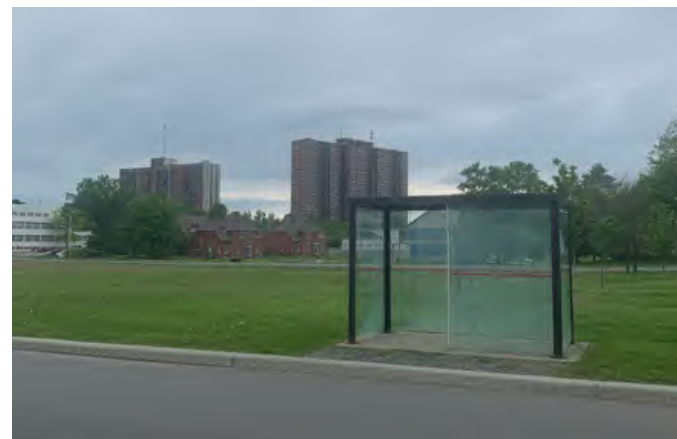
FIGURE 40. EXISTING BUS SHELTER ON HOWLETT STREET Source : Stantec
