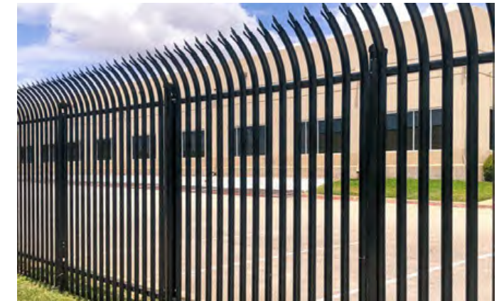
FIGURE 146. SECURITY FEATURE, HIGH SECURITY STEEL PALISADE FENCE Source: Ameristar Assa Abloy
