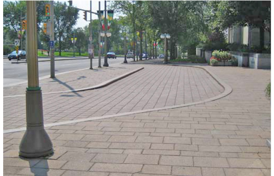
Figure 44: Example of unit paving pattern changes at driveways
